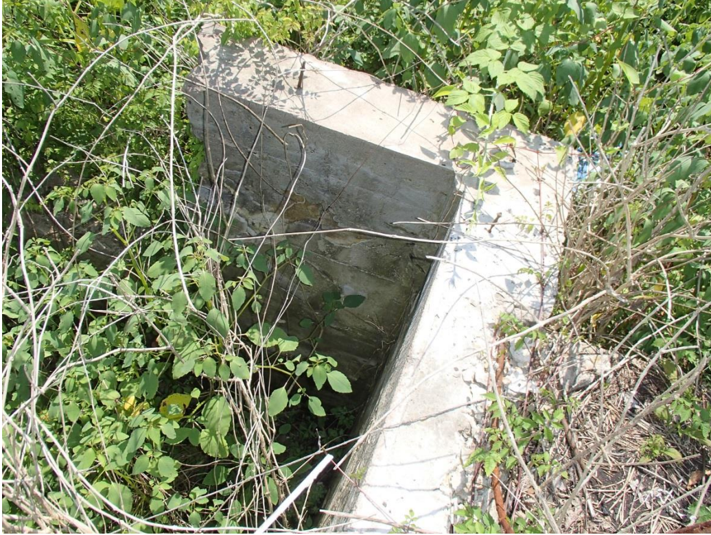
Figure 3-7. Historic foundation detail.
