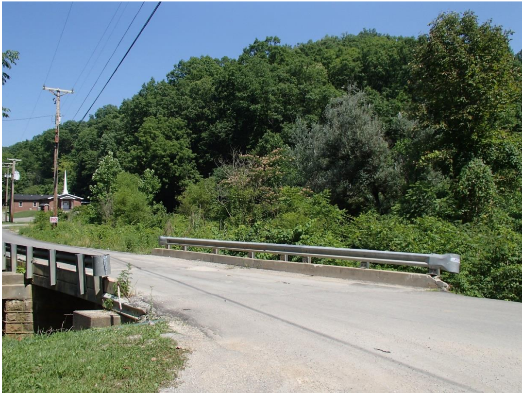
Figure 1-4. General project area, north side of KY 2021, looking northwest.
