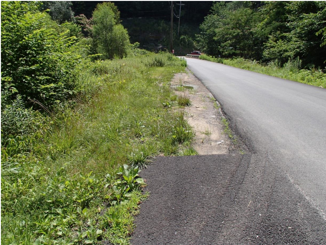
Figure 3-14. View of APE ROW extension, north side of KY 2021, looking east.
