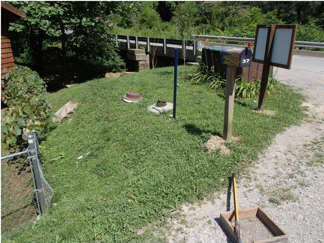
Figure 3-10. View of APE, proposed ROW extension, south side KY 2021, at Beech Oak Road intersection.
