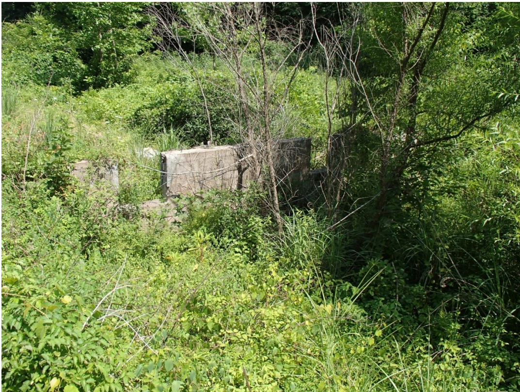
Figure 3-8. View of APE, historic foundation, looking southwest.
