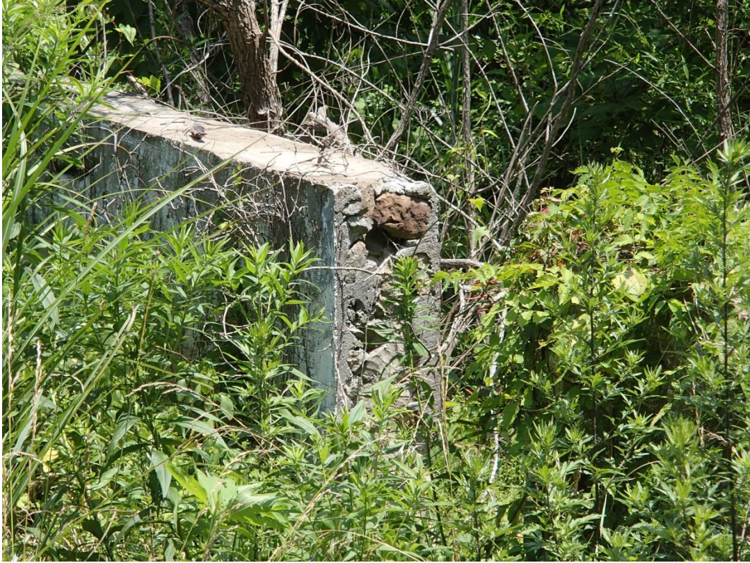
Figure 3-9. Historic foundation detail.
