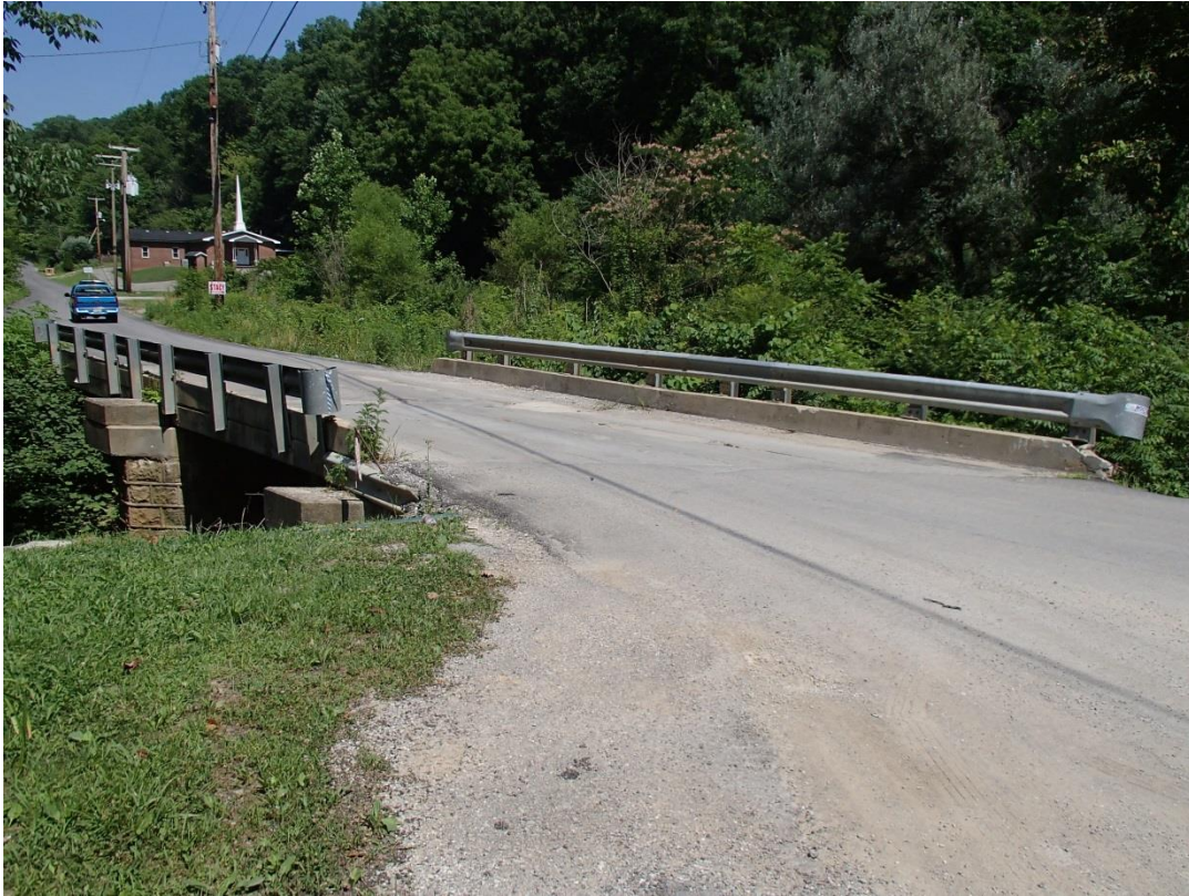
Figure 3-3. View of existing KY 2021 Bridge, looking northwest.
