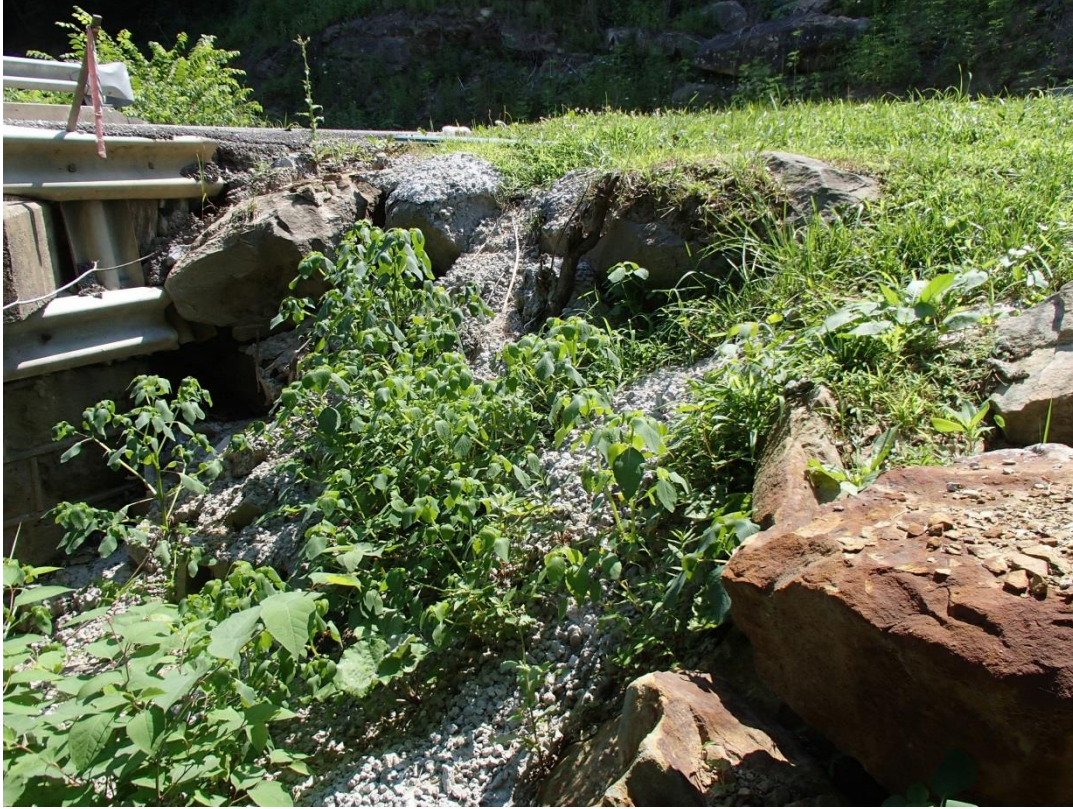
Figure 3-11. View of APE proposed ROW extension, south side of KY 2021, eastern end, looking east.
